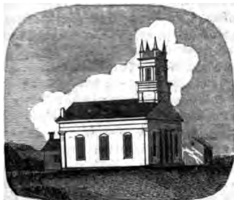
St. Stephen's Church, North Castle.
